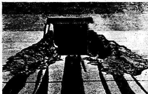
Fig. 9. Erosion of faced junction after passage of one flood.
